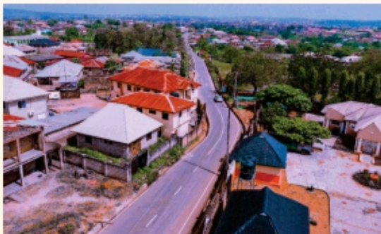
A completed road by Adeleke administration in Ikire, Irewole local government area of the State.
