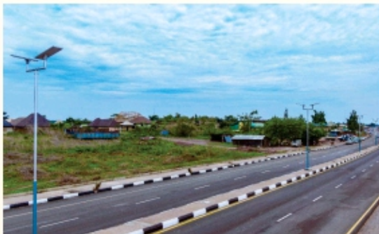
Completed Osogbo-Ikirun-Kwara boundary road inherited from the previous administration.
