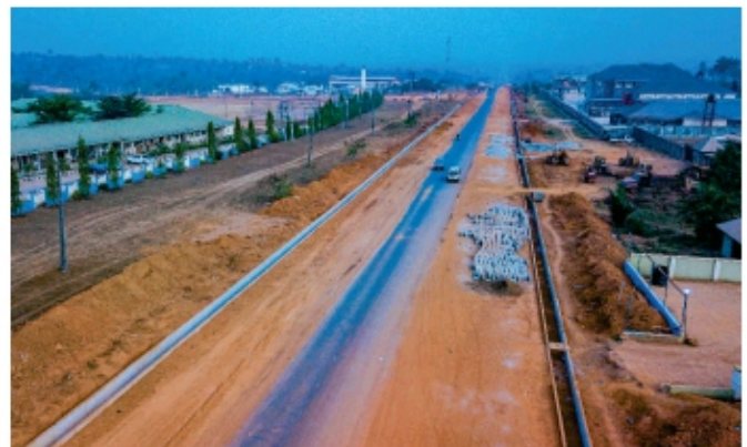
Ongoing dualisation of Akoda-Okegada road in Ede
