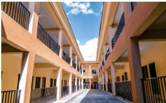
Inside view of the Health sciences faculty offices and lecture rooms.
