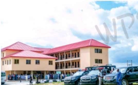
Outside view of the completed Office and lecture rooms at the Health Sciences faculty of Osun State University, Isale-Osun, Osogbo.
