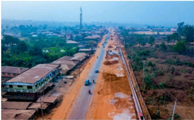
Another section of the ongoing Akoda-Okegada road.
